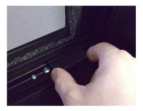
Wearing gloves and/or using suction cups, lift the glass into place and rest the bottom edge on the two setting blocks and up against the rubber seal on the inside of the window jamb. Gently tilt the top of the glass into place making sure it is centered in the opening.
